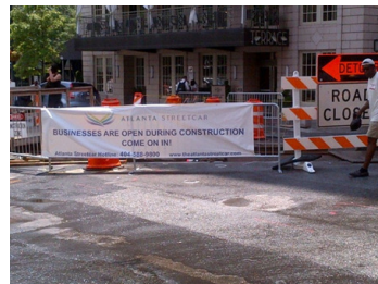
Businesses remain open along the Streetcar route during construction.
