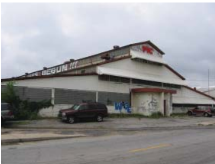
This building is one the identified historic buildings along the BeltLine.
