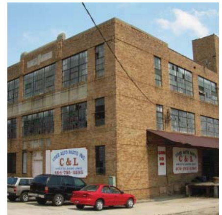
The John Fulker building is one the identified historic buildings along the BeltLine.
