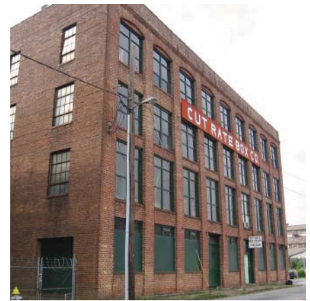
The Cut Rate Box is one the identified historic buildings along the BeltLine.
