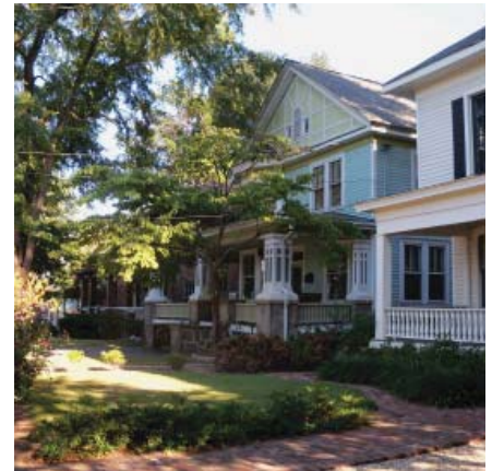
These homes are classified as Low Density Residential in the existing land use inventory.
