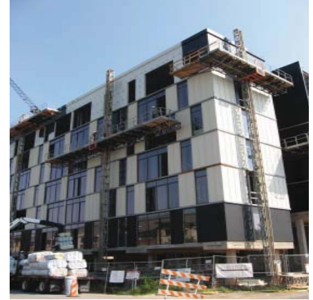
Board Stone multi-family building under construction on Marietta Street, NPU E.
