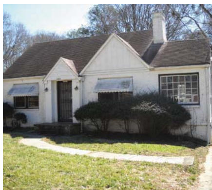
This house on Allegheny Street was purchased with NSP funds, NPU T.
