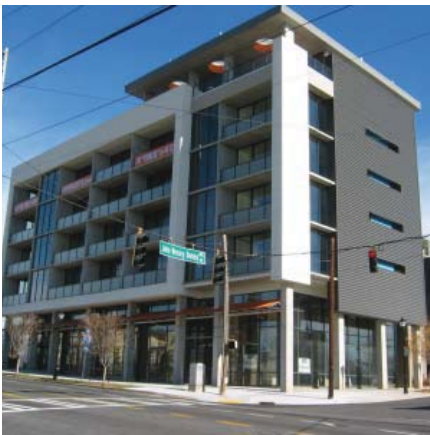
Tribute Lofts in the Eastside TAD has 20% affordable units.
