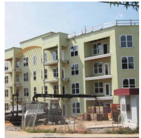
Rental housing units under construction.
