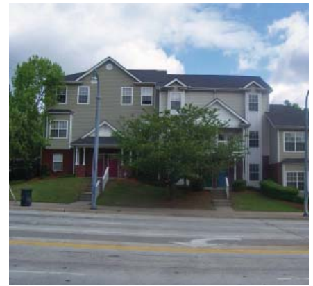
Townhomes in Mechanicsville built by a CDC, NPU V.
