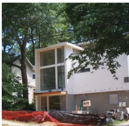
New Single family home construction in Candler Park, NPU N.
