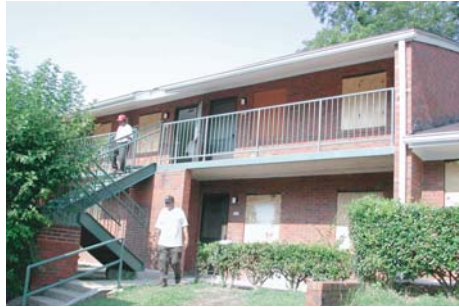
McDaniel Glenn Annex before renovation
