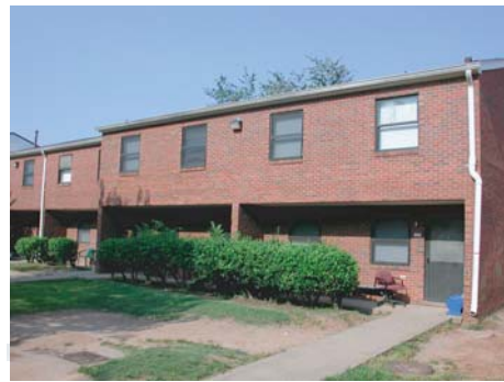
McDaniel Glenn Annex before renovation
