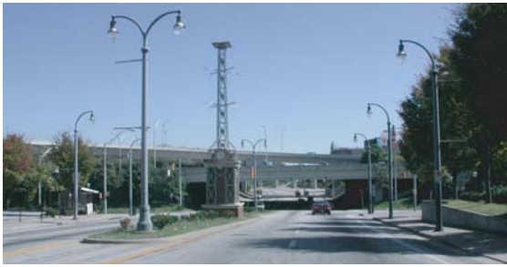
Retail area before improvements
