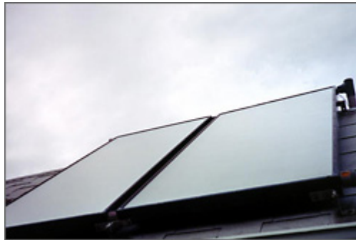
Figure 3: Flat Plate Solar Collector (NREL, 2007)
