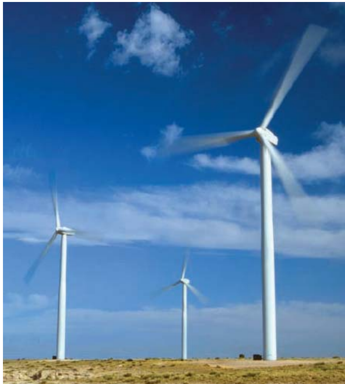
Figure 10: GE 1.5 MW Wind Turbine
