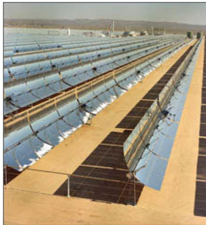
Figure 4: Concentration Collectors (NREL, 2007)
