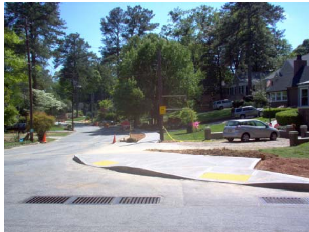
Construction Nearing Completion!
