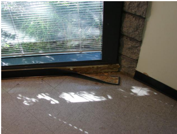
Damage to window frame and possible mold at APD Zone 1 Precinct
