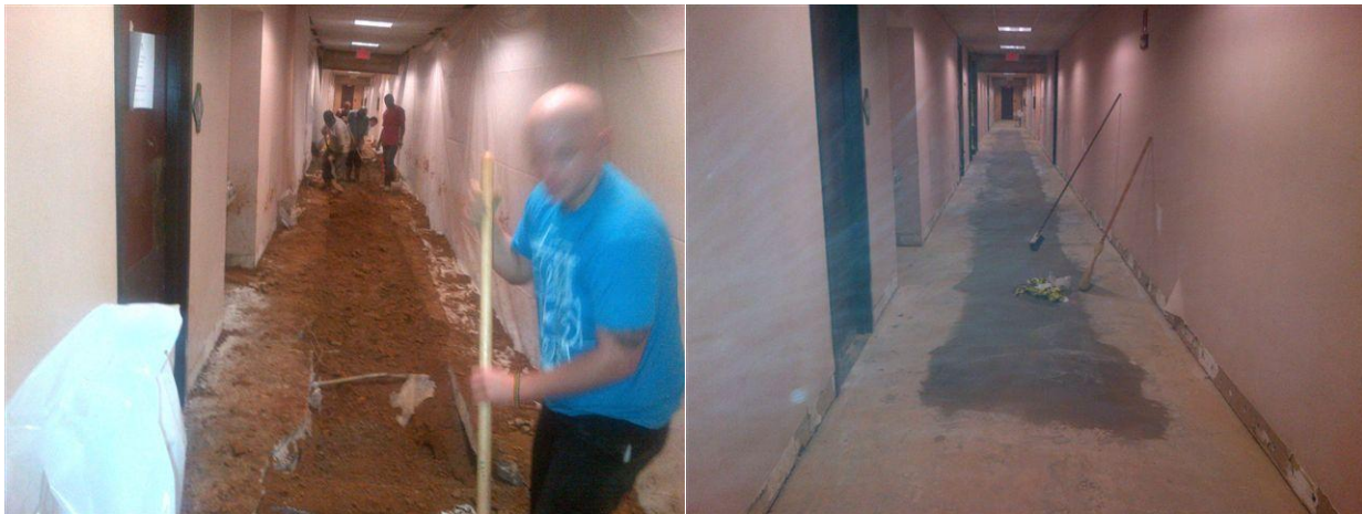
Before and after a City Hall Utility Repair
