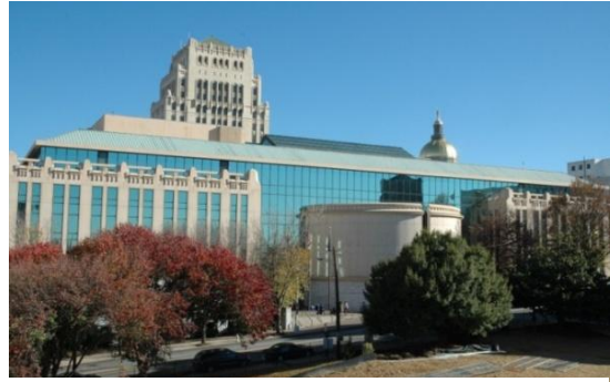
Trinity Ave. Entrance of Atlanta City Hall
