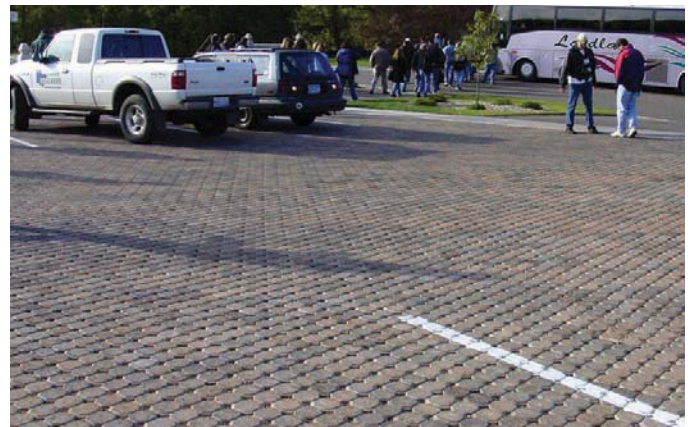
Pervious paving allows stormwater to percolate into the ground
