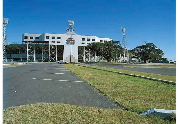
Eco-sensitive paving option at Ladd Stadium in Mobile, AL includes pervious pavement and bioswales
