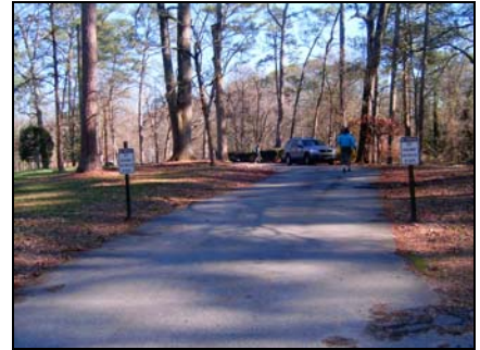
Existing Asphalt Driveway
