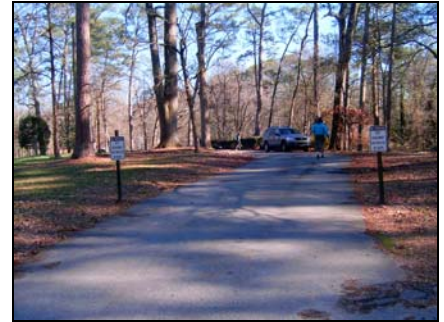
Existing Asphalt Driveway
