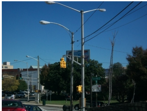
Cobra Head Street Lights at Spring Street and Trinity Avenue
