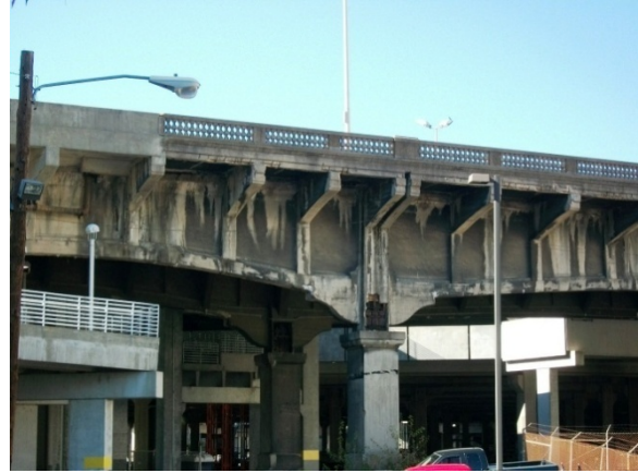
Spring Street Bridge
