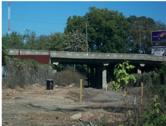
Edgewood Road Bridge over abandoned railroad
