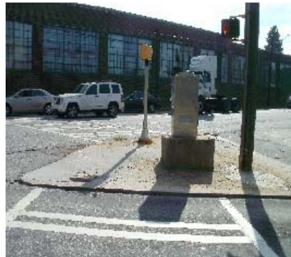
Missing ADA Ramp Location
