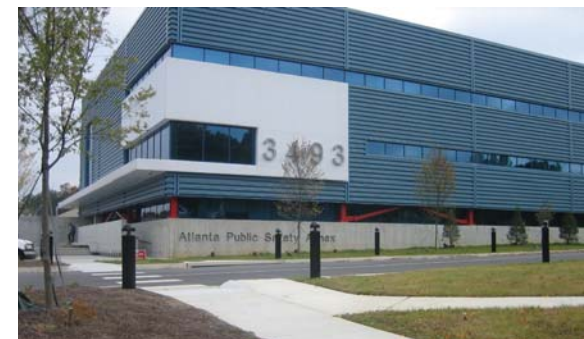
PUBLIC SAFETY ANNEX AT ATLANTA INDUSTRIAL PARK
