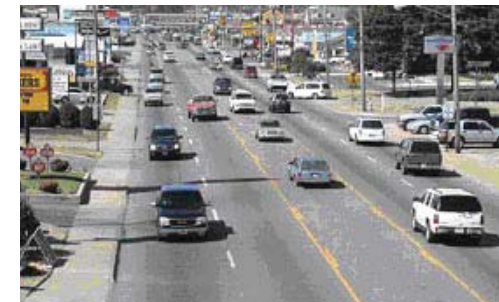
EXAMPLE OF POOR ACCESS MANAGEMENT
