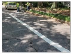
Retroreflective Striping (typical) Typical Dimensions: 4"W Estimated Cost: \$3/LF
