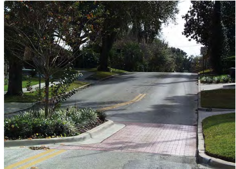
Center Island narrowing on a street
