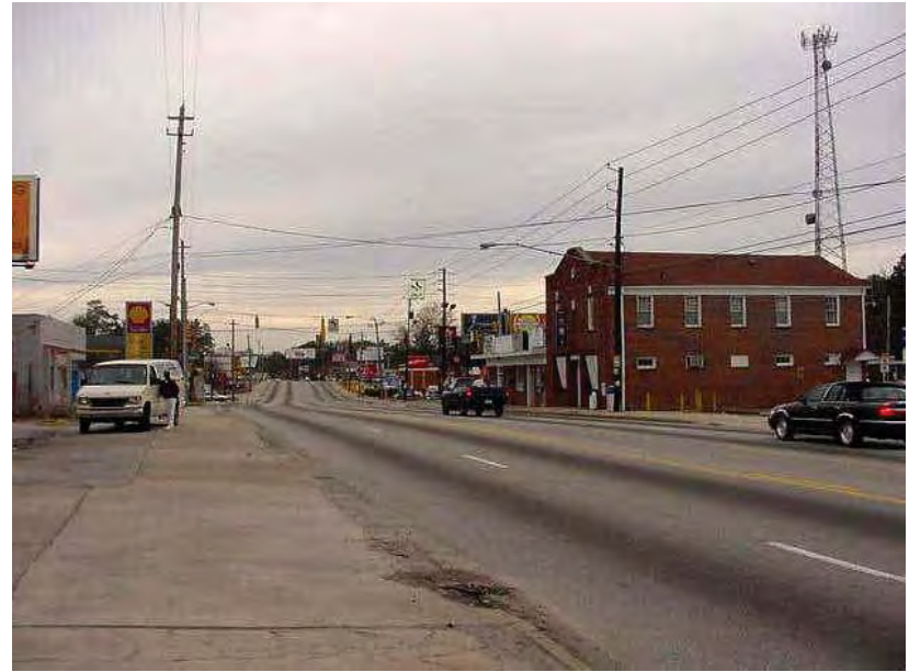
Campbellton Road at Fairburn Road - Before
