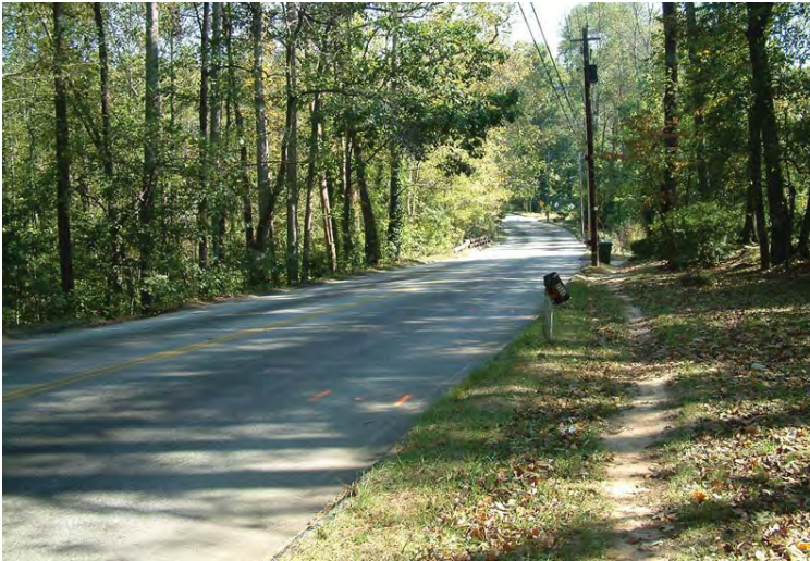
Two lane section of Campbellton Road
