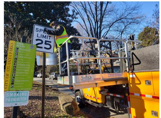
Image: Installation of new 25 mph signage
