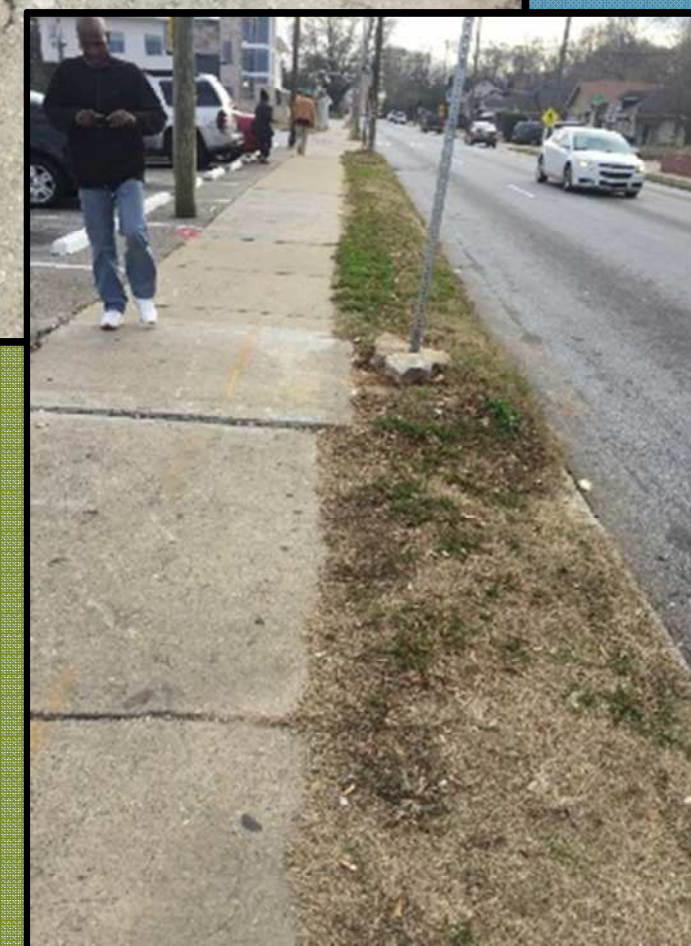
Existing Sidewalk along Lowery
