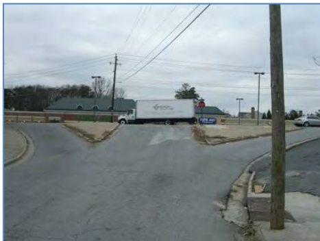
Steep grade on Emery Street approaching intersection with Collier Road
