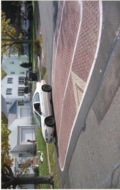
Speed tables are usually preferable to speed humps in that they are more accommodating to delivery and emergency vehicles, yet they also provide a cue to use lower speeds.
