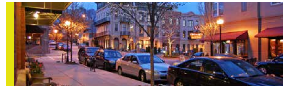
From top to bottom: Views of Downtown, Midtown, Decatur and Glenwood Park in Atlanta, GA.
