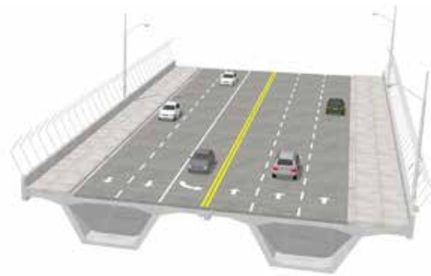
Capitol Avenue Bridge Existing Condition
