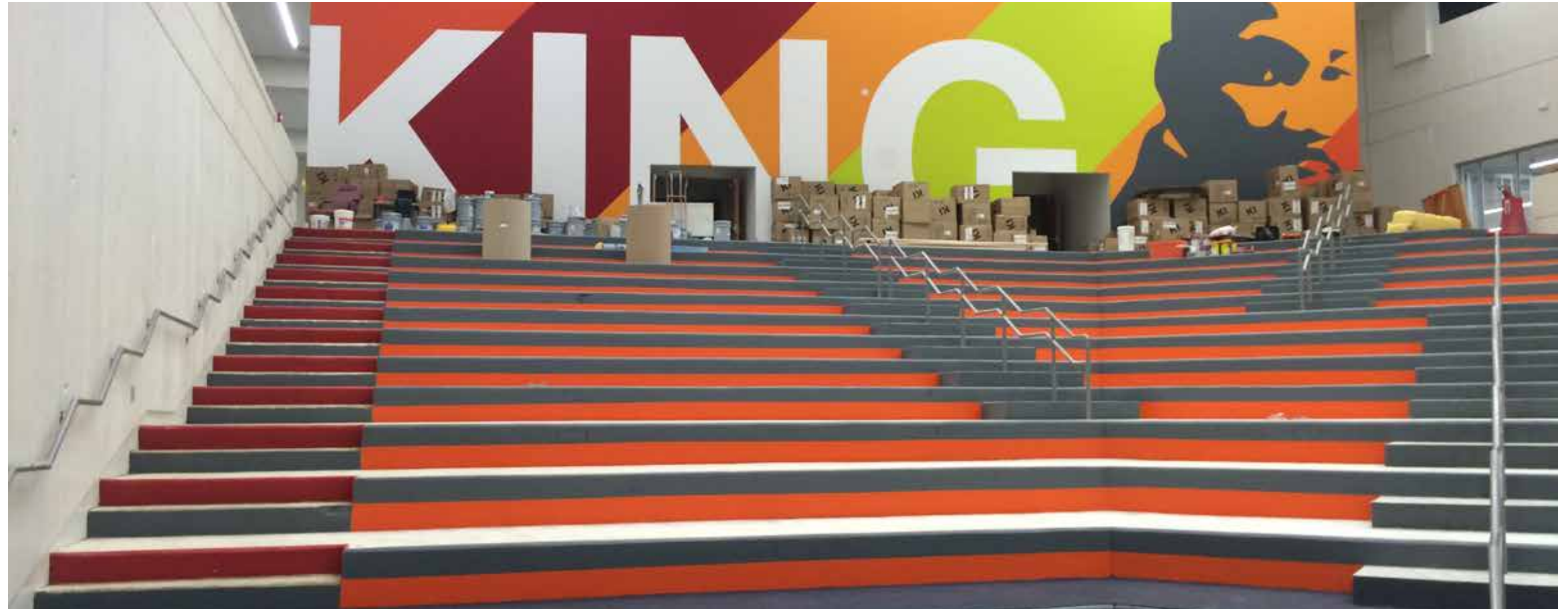
King Middle School under renovation, Atlanta, GA.
