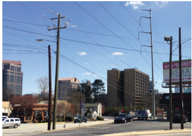
The burial of low voltage utility lines with redevelopment can make a large impact of Roswell Road's streetscape. While the high voltage lines are extremely costly to move, an art program on these poles may be considered.
