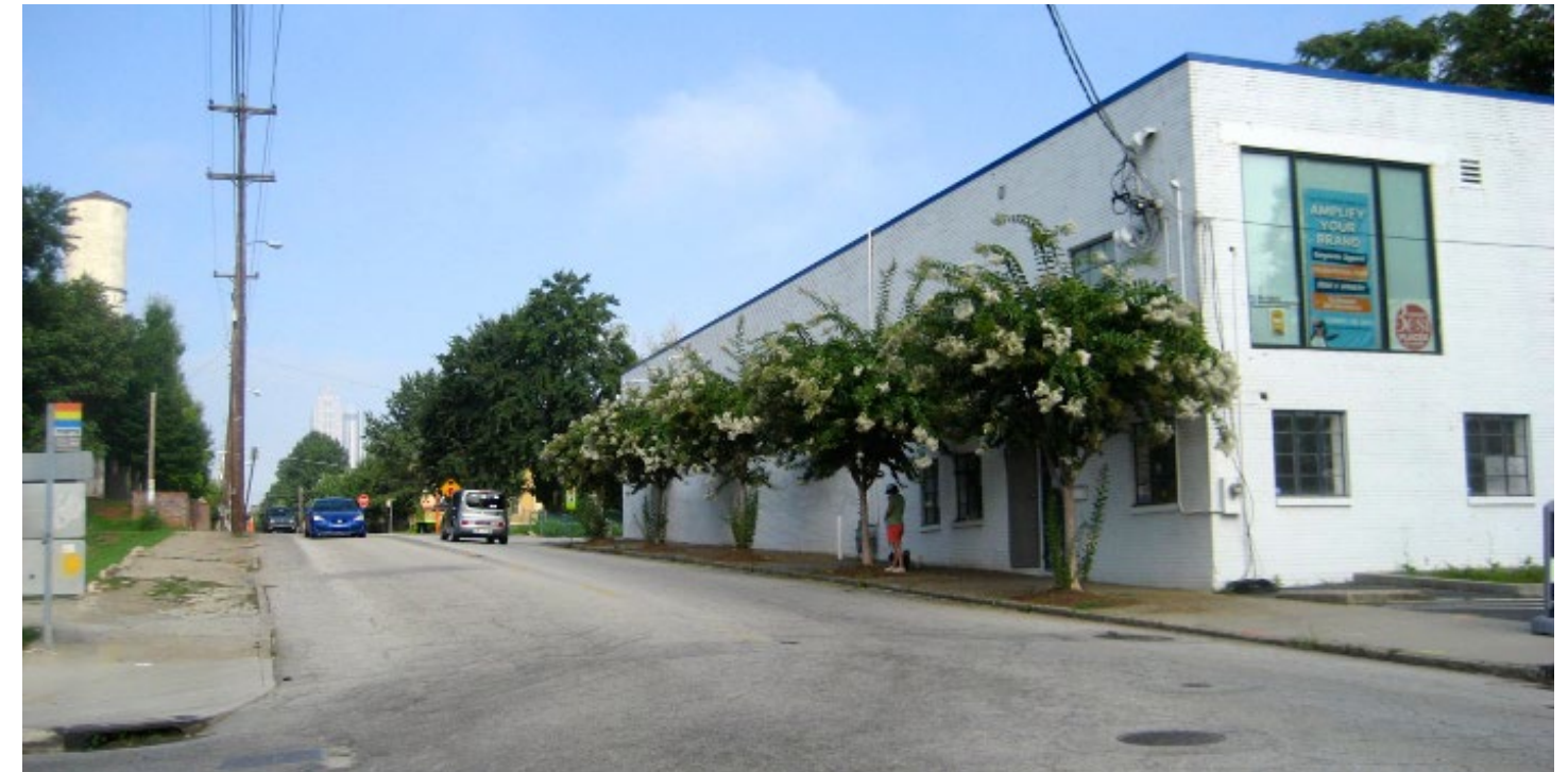
Irwin Street/Lake Avenue @ Krog Street: Existing
