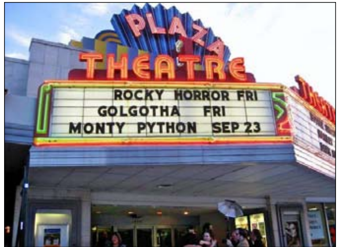
Briarcliff Plaza dates from 1939 and was renovated in 1982
