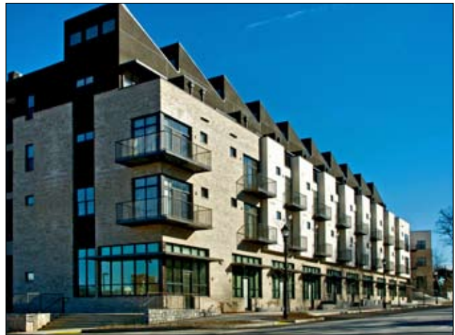
Buildings on North Highland Avenue should be three stories at the street, but may step up behind the front facade (courtesy Smith Dalia Architects)
