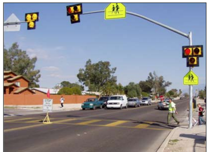
“HAWK” signals only turn red when pedestrians need to cross the street
