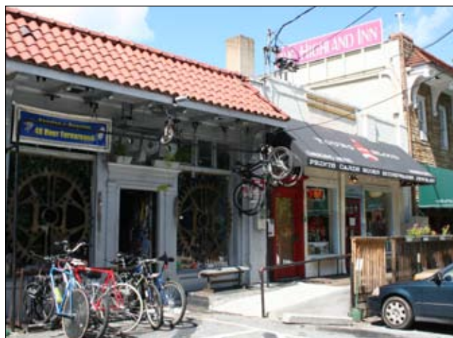
Historic commercial buildings were built touching each other on the sides to create a continuous street wall
