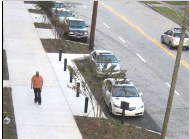
In the Old Fourth Ward the curb was moved in on Ralph McGill Boulevard to create new on-street parking
