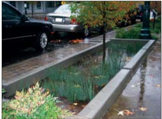
Bio-swales along stormwater to slowly infiltrate into the ground, while also providing greenery
