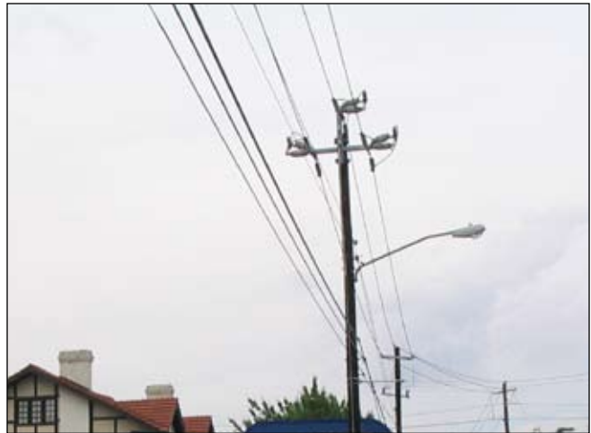
Although costly, burying utility wires with redevelopment can significantly improve neighborhood aesthetics
