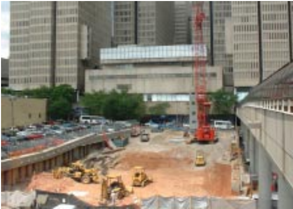
InterPark Garage at Peachtree Center
