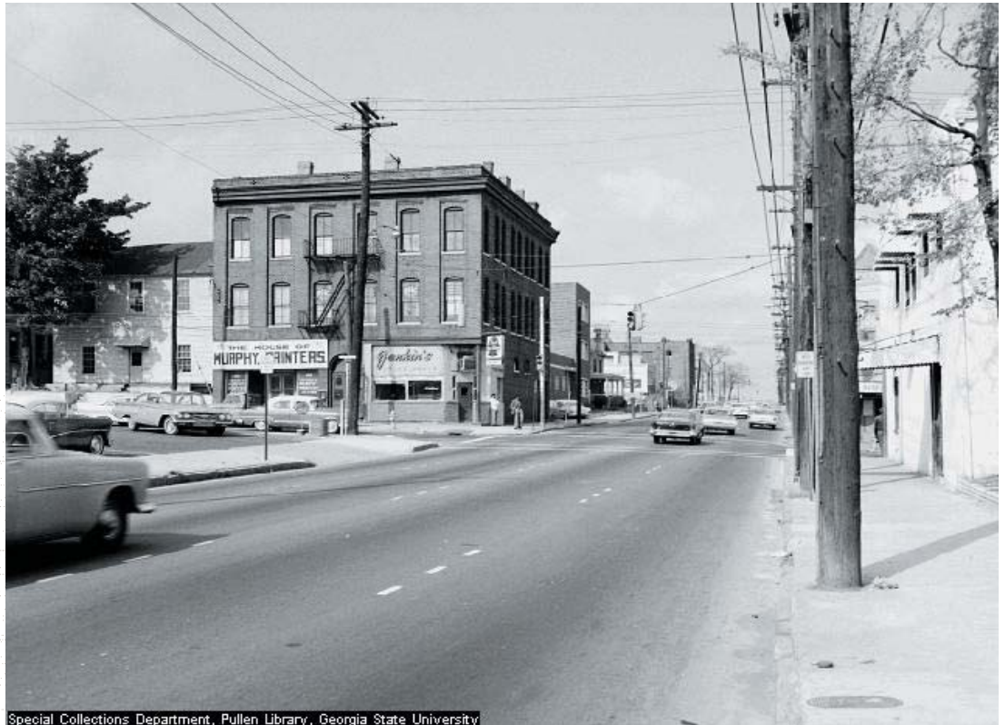
Figure 1.0: Rucker Building from Piedmont Avenue
