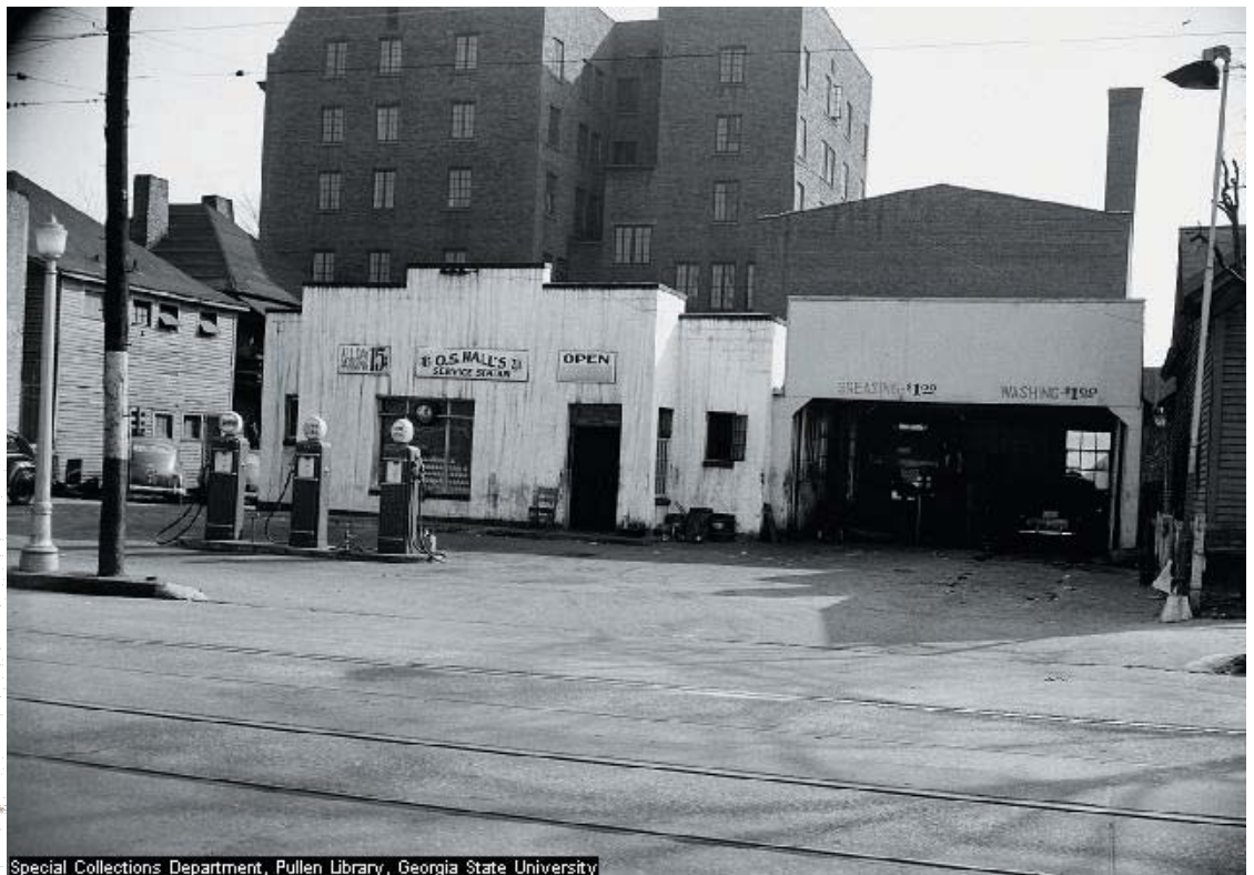
Figure 3.0: Hall's Service Station
