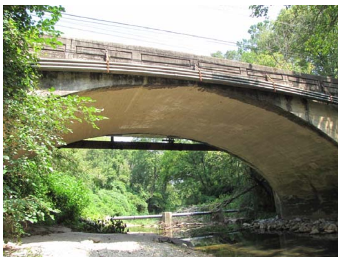
Figure 2.1e: Proctor Creek at the Johnson Road Bridge
