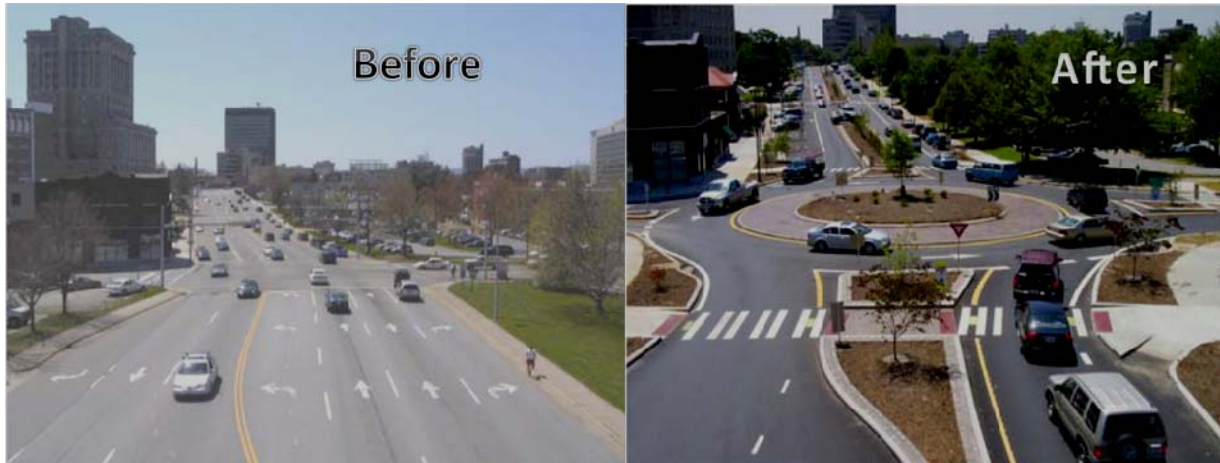
Figure 2.3b: Roundabout Used as A Gateway in Asheville, North Carolina
