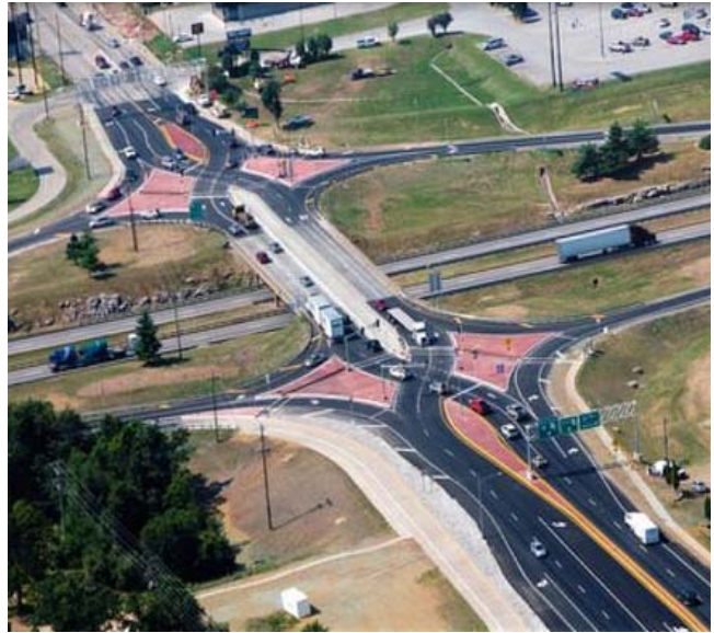
Figure 2.3a: Diverging Diamond Interchange, Springfield, Missouri
