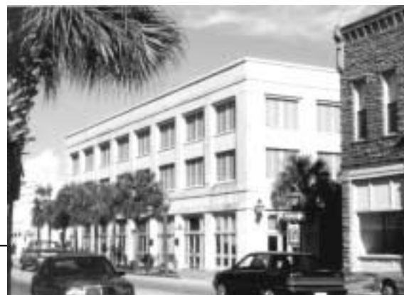
Figure 5: 4 Parking decks can be designed to look like buildings, such as this one in Charleston, SC.
