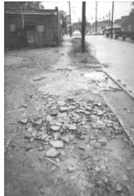
Figure 4: 1 Broken sidewalks along Metropolitan Avenue discourage walking from residential areas to the Village.
