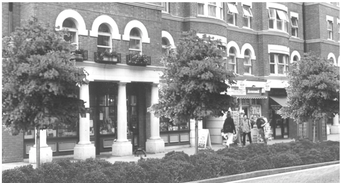
Figure 7: 6 The streetscape treatment along Moreland Avenue will include a ten feet wide planting area between the street and the sidewalk planted with shrubs and trees, as well as a ten feet wide clear zone.
