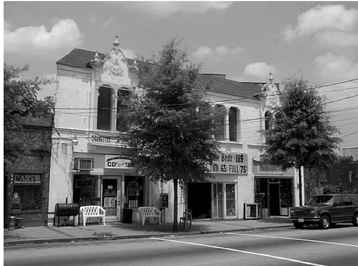
Figure 8: Madison Theatre along Flat Shoals Road. 1998.
