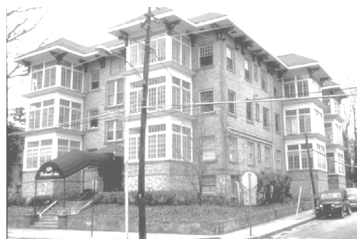
Figure 2: 8 Some workshop participants would like 1920s-style apartment buildings along Moreland
