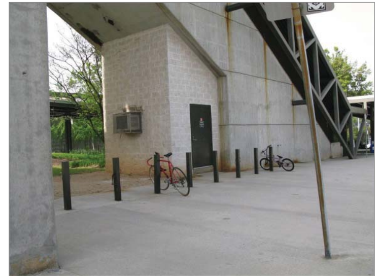
Bicycle Facilities in the MARTA Parking Lot
