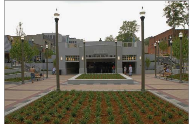
The Decatur MARTA Station received LCI funding to renovate the station.
