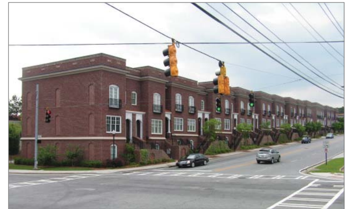
Townhomes were developed on surplus MARTA parking at the Chamblee Station.
