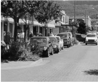
On street parking and landscaped bulb outs slow down vehicular traffic by narrowing the street in Seaside, Oregon.
