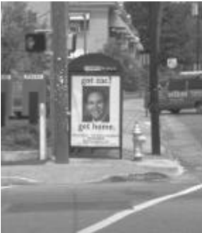
Sidewalk amenities combined with a narrow sidewalk create dangerous conditions at this corner of the intersection.
