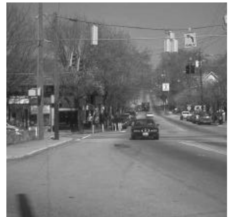
This travel lane is unnecessarily wide.
