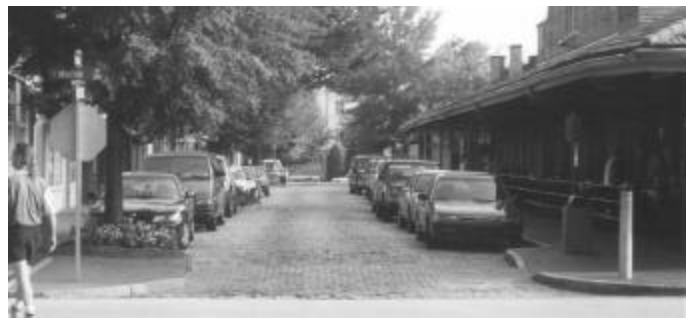
Bulb-outs accommodate on-street parking and shorten the crosswalk distance across the street here in Raleigh, North Carolina.
