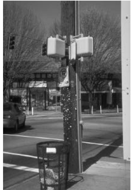
Utilities on the sidewalk cause visual clutter.
