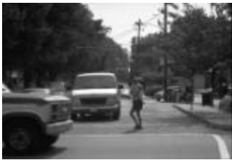
Existing crosswalks fail to draw attention to pedestrians.
