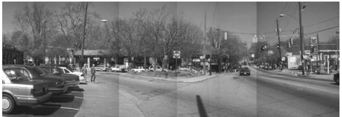
Wide travel lanes and an insignificant gateway triangle characterize the existing Virginia Avenue and North Highland Avenue intersection.
