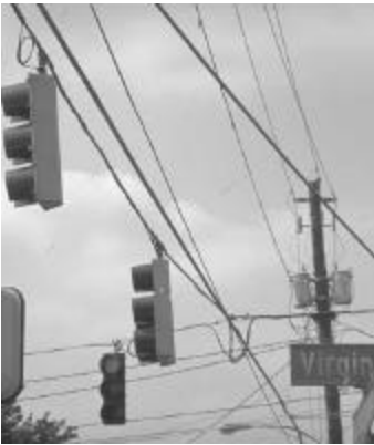
Inadequately timed traffic lights.
