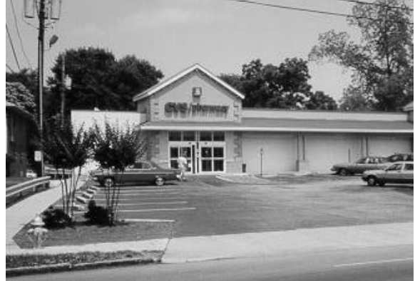
Parking for developments built over the past thirty years has placed parking between the building and the sidewalk.
