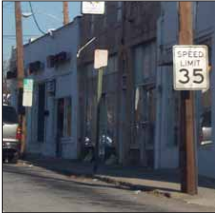
Utilities should either be removed from the sidewalk or buried as part of new development
