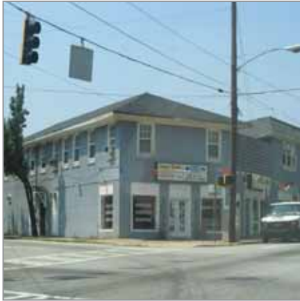
A commercial building in Lakewood Heights
