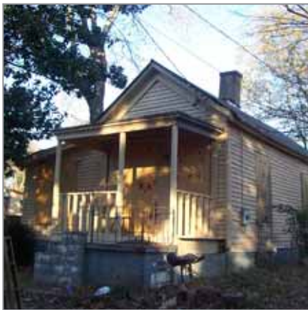
"Dilapidated" building condition
