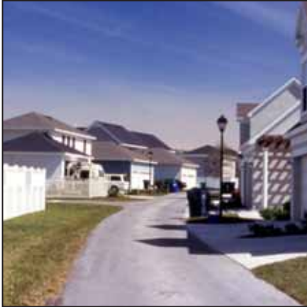
Rear lanes are a form of access management that can reduce curb cuts on streets
