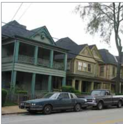
Queen Anne homes in the Sweet Auburn Historic District in Atlanta
