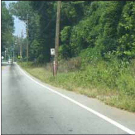
The extra curb and gutter space along Jonesboro Road could be confused with a bicycle lane
