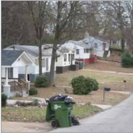
Several deteriorated Minimal Traditional style homes line Schoen Street
