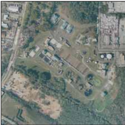
The South River Water Reclamation Facility is located along the South River, off Cleveland Avenue.
