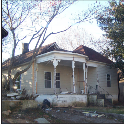
Substandard building conditions are common in the Study Area
