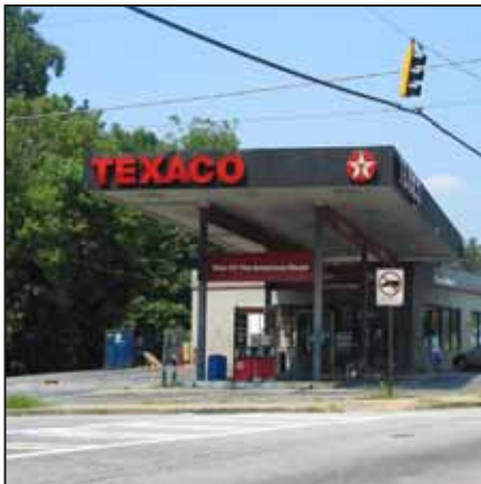
This gas station at the corner of Hutchens Road used to be a passenger rail stop
