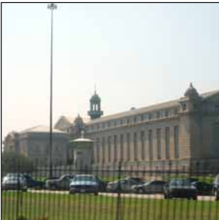
With readily available rail access, the Federal Prison is an ideal location to maintain industrial activity
