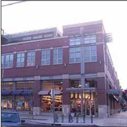
The Lakewood Heights parking deck should be screened from the street by liner uses, such as ground floor retail and above-shop offices
