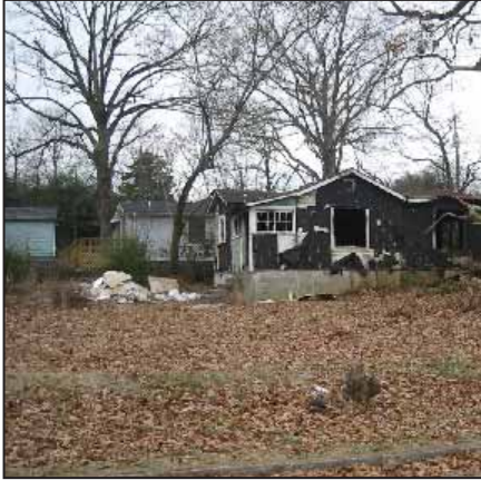
Adverse environmental conditions, such as illegal dumping and structural deficiencies, are also indicators of distress and blight
