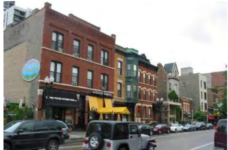
Horizontal Roof Rear Parking Brick with Storefronts Continuous Buildings
