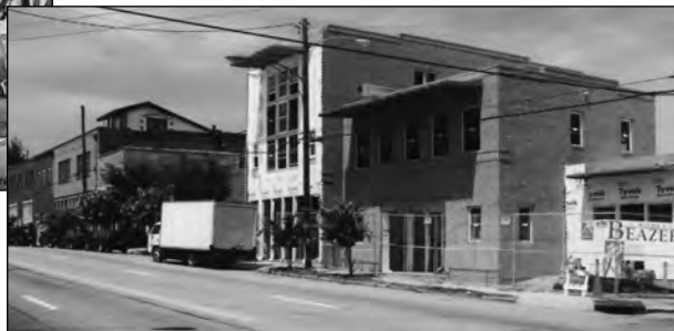
Plans were revised and the actual construction better fits the industrial character of the neighborhood with flat roofs similar to buildings in the same block.
