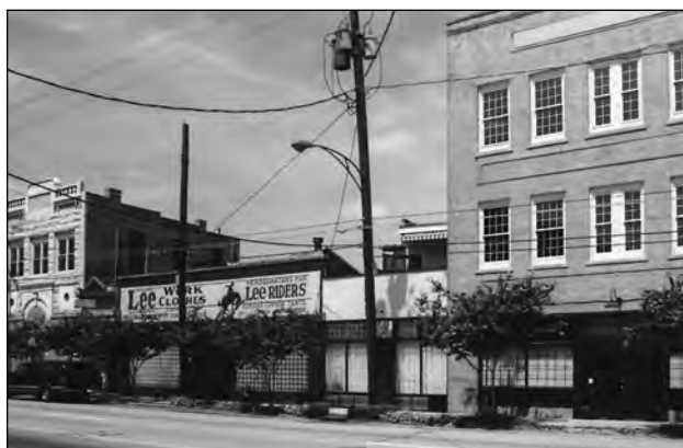
Renovated buildings along Peters Street.
