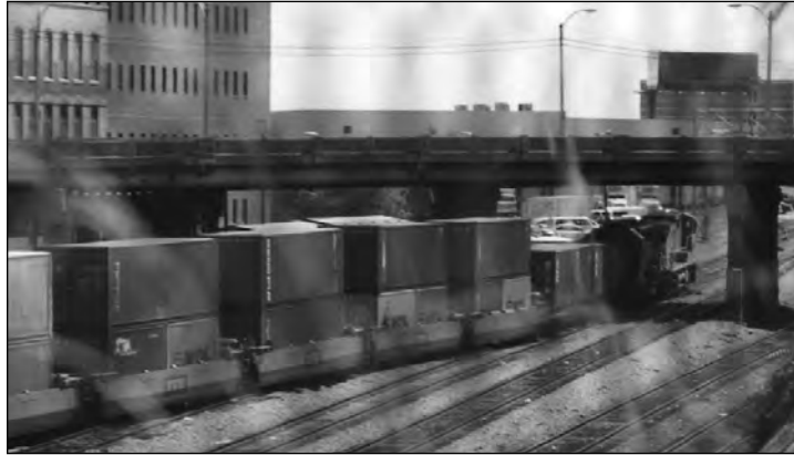
A train with double-stacked containers passing under the Peters Street Bridge, which is supposedly of "inadequate height for modern rail needs."
