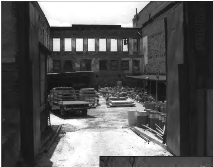
Houseparts, a decorative arts manufacturer and distributor, occupies several buildings on Whitehall Street
