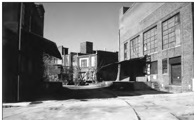
Looking south along the railroad spur at Mangum Street.
