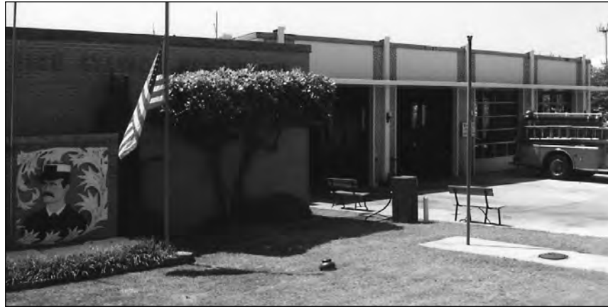
Fire Station No. 1 on Elliott Street.
