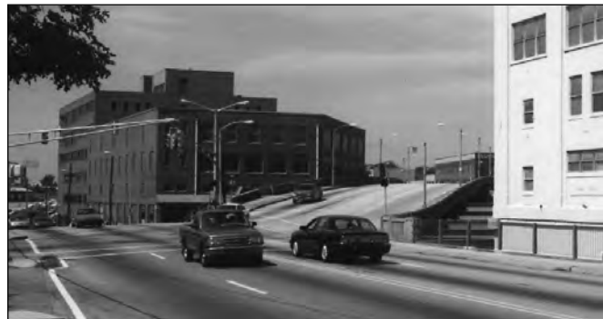
Spring Street and the Peters Street bridge.
