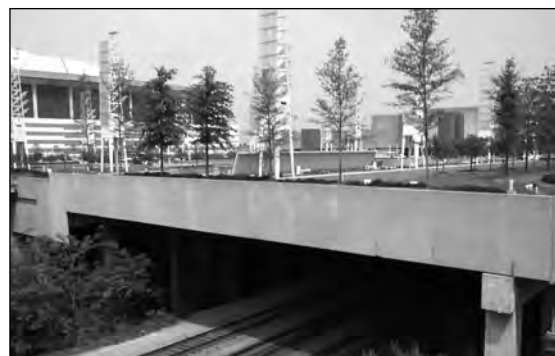
The plaza outside the Georgia Dome and Georgia World Congress Center is an example of effectively building pedestrian spaces over support, service and parking spaces.
