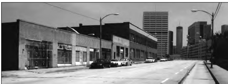
The present, pedestrian-scaled Peters Street bridge.
