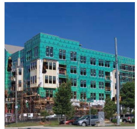
Multi-Family building under construction.
