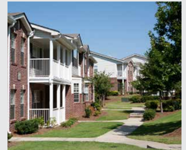
MULTIFAMILY HOUSING @ THE VILLAGES AT CARVER IMAGE VIA ATLANTA HOUSING AUTHORITY
