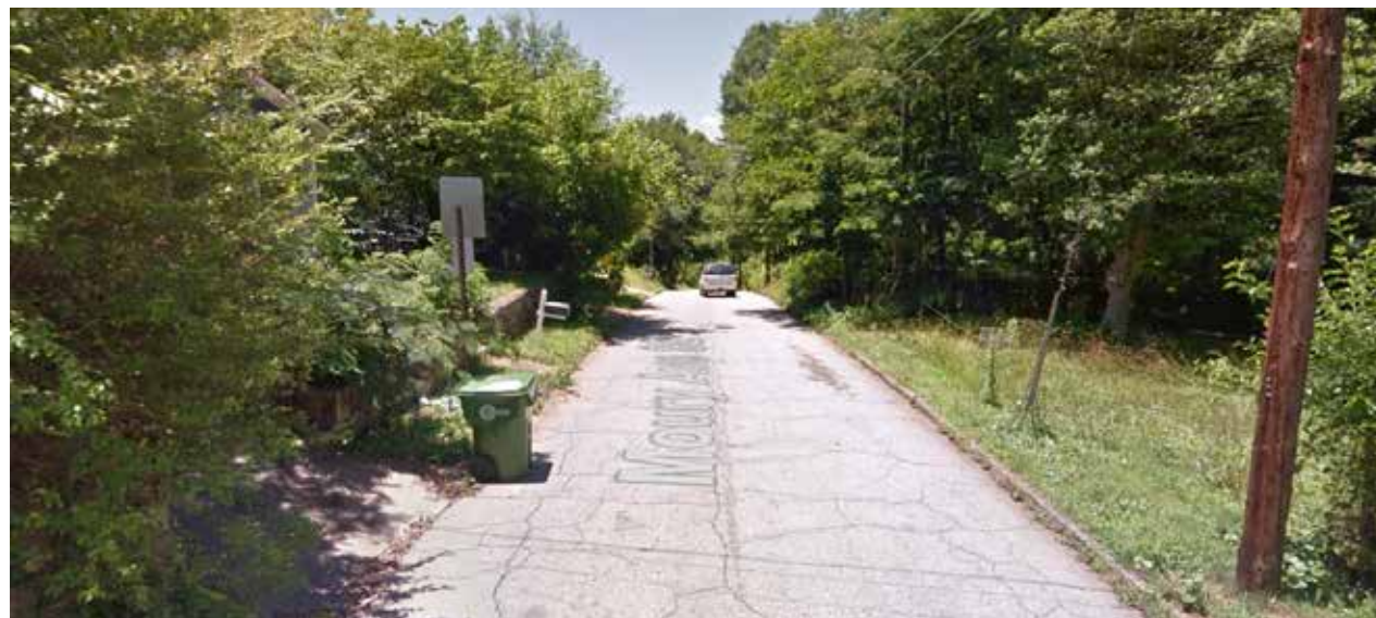
MOURY AVE - NO SIDEWALKS, OVER-GROWN TREES, UNSAFE CUES IMAGE VIA GOOGLE STREETVIEW
