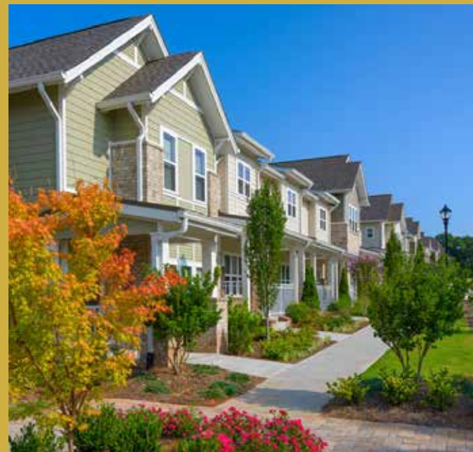
EDGEWOOD RETREAT TOWNHOME DEVELOPMENT MANAGED BY THE ZEIST FOUNDATION IMAGE VIA SMITH DALIA ARCHITECTURE
