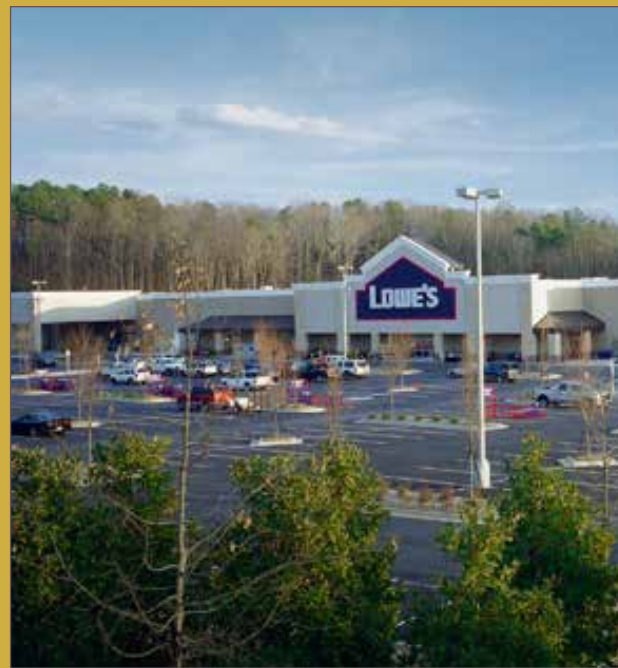
LOWE'S AT CAMP CREEK MARKETPLACE IMAGE VIA COLLINS AND ARNOLD CONSTRUCTION
