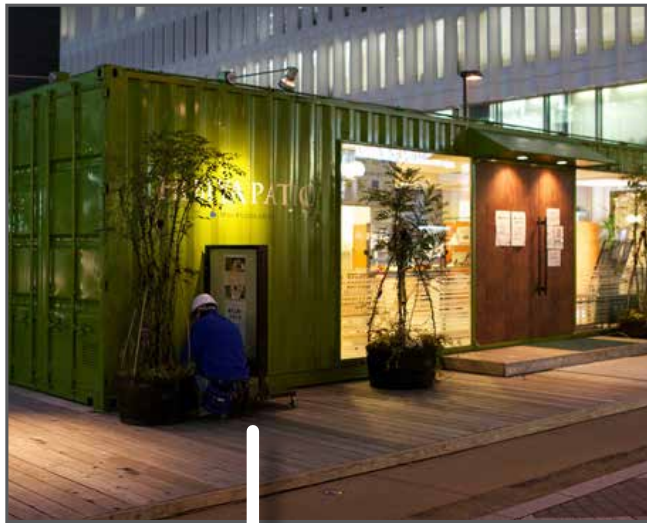
TEMPORARY GALLERY SPACE WITH DECK BUILDOUT
