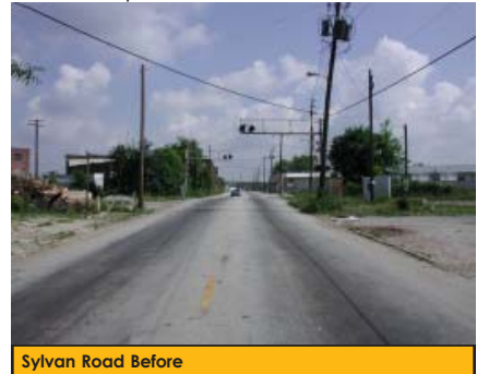
Figure 10.1: Sylvan Road Before and After Improvements
