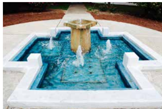
Smith Park Foundation Renovation Before and After Images via MLPA.org
