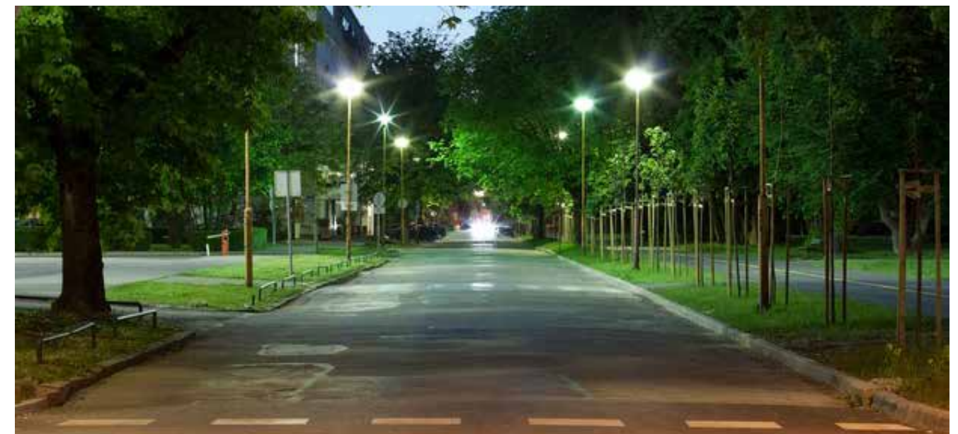
LED lighting is more illuminating and has become less expensive for street lighting improvements. Image via brandonindustries.com
