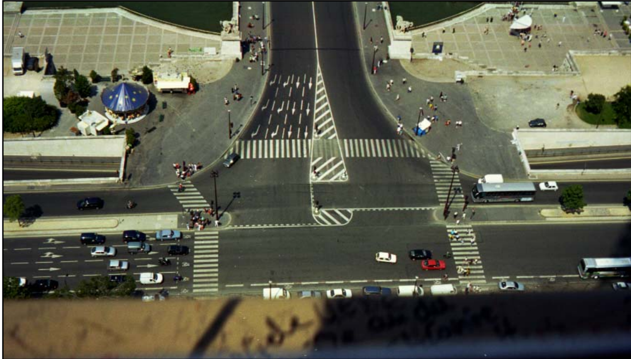
As shown in this picture, it is recommended that medians provide pedestrian refuges at intersections
