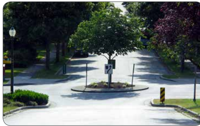
Mini-Traffic Circle with integrated bulbouts
