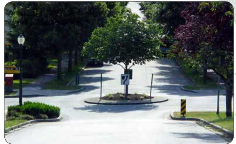
Bulbouts used in conjunction with Mini-Traffic Circle
