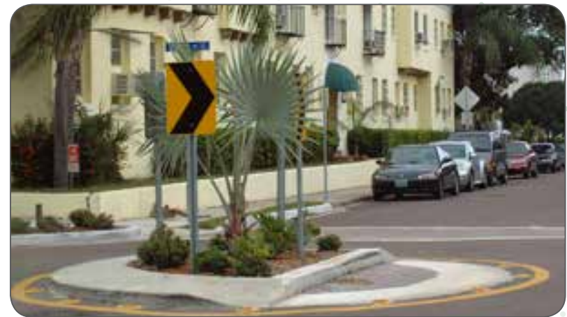
Half Traffic-Circle used at T intersection in Winter Park, FL
