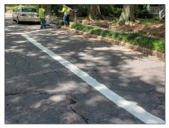
Retroreflective Striping (typical) Typical Dimensions: 4"W Estimated Cost: \$3/LF
