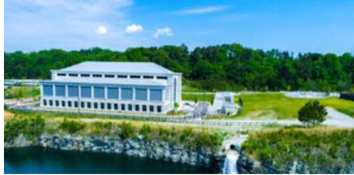
Westside Water Supply – Pump and Outfall Photo Courtesy of Department of Watershed Management
