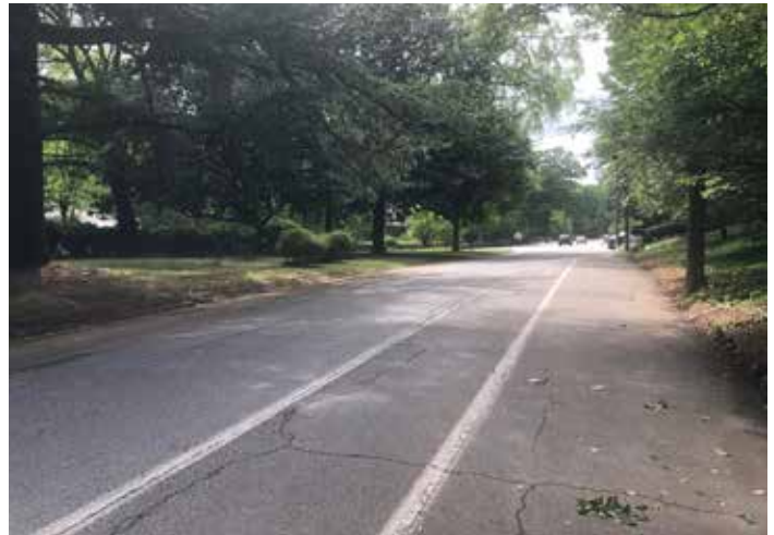
Existing Peachtree Battle Avenue travel lane, bicycle lane, and parking lane.
