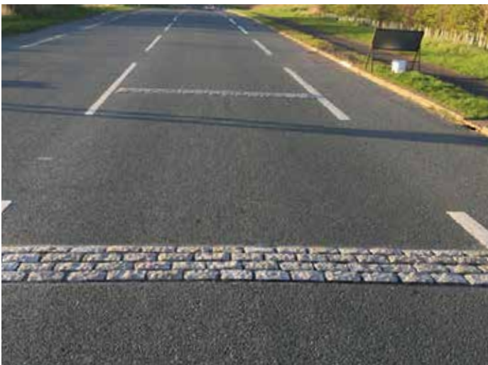
Rumble strips are textured surfaces in the roadway that alert drivers. (courtesy Quicksetts)
