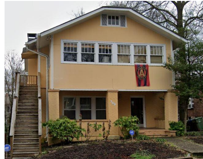
Stacked Duplex One unit on top of another. Square or vertical proportions.
