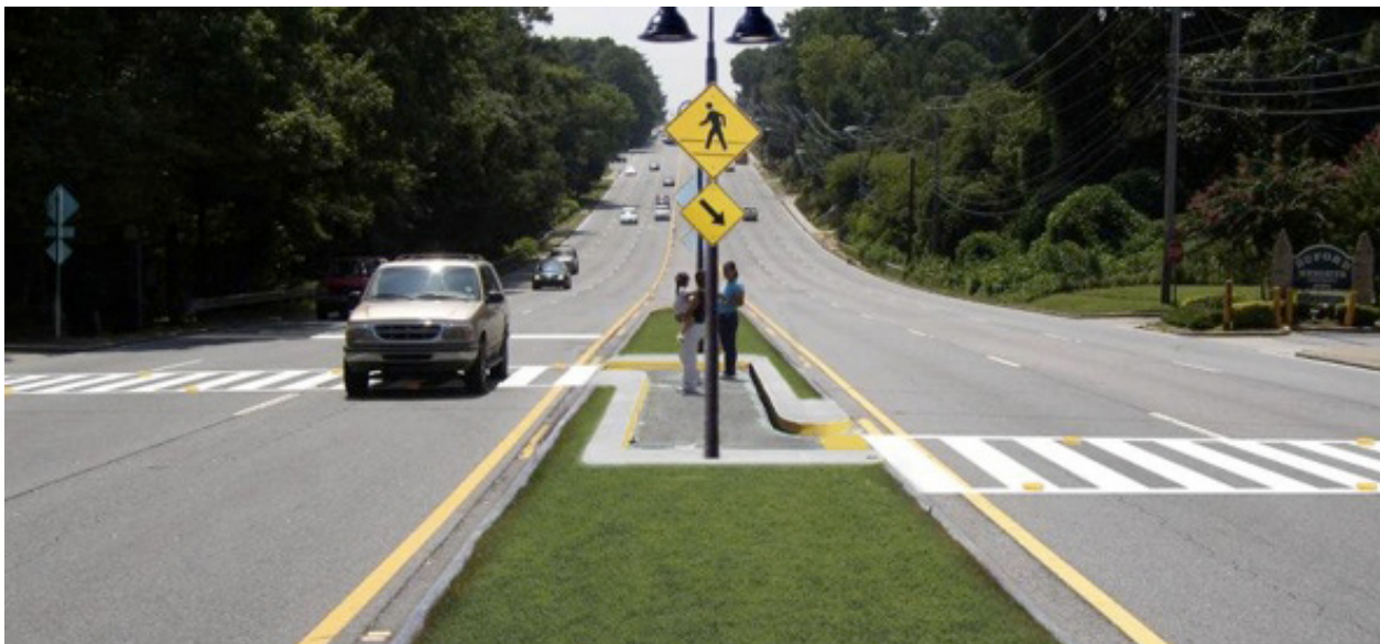
Staggered crossing with refuge island, Buford Highway
