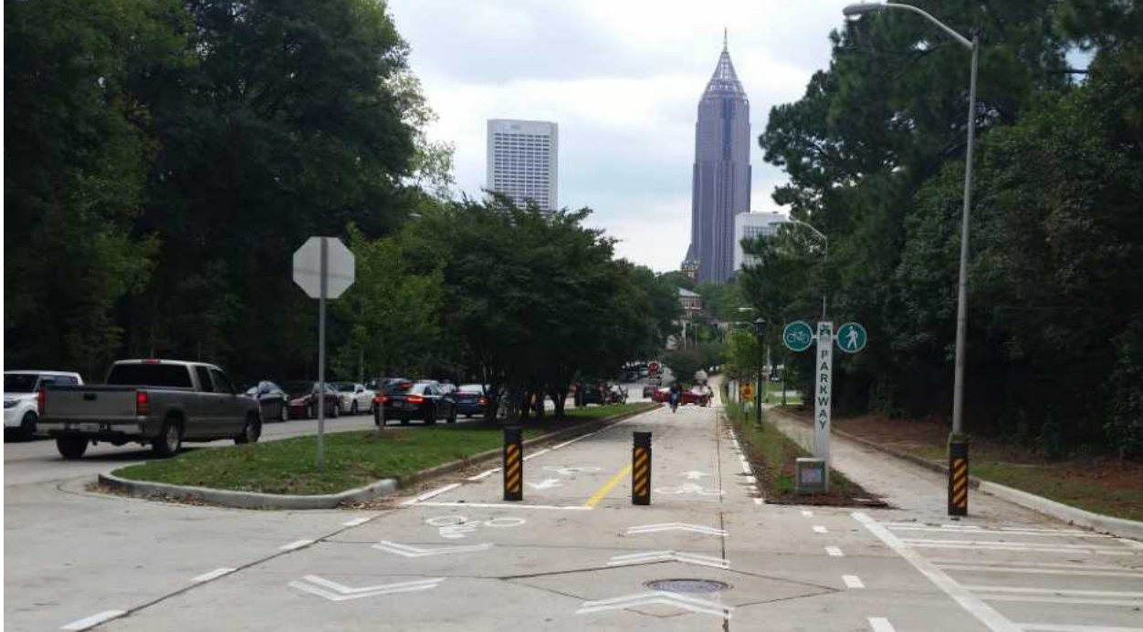
A two way protected cycle track at Tech Parkway .
