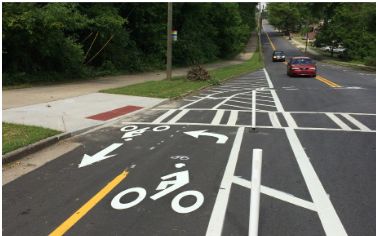
The Westview Drive two-way protected bike facility was installed to create a network with an existing multiuse path
