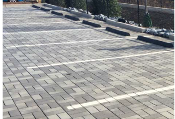
Permeable pavers used for parking lot
