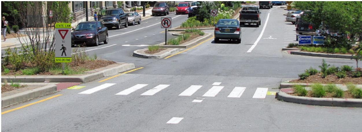
Curb extensions and medians make crossing four-lane streets safer and more manageable to cross (Credit: Dan Burden)
