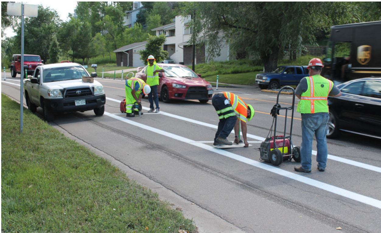
A four lane street in Boulder, CO was reduced to a single lane in each direction, a center turn lane, and a protected bike lane with bollards.
