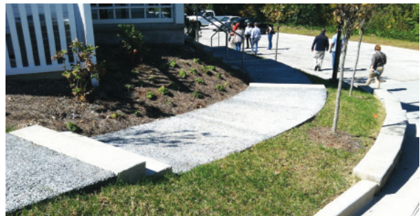
Pervious concrete sidewalk in Chattanooga, TN
