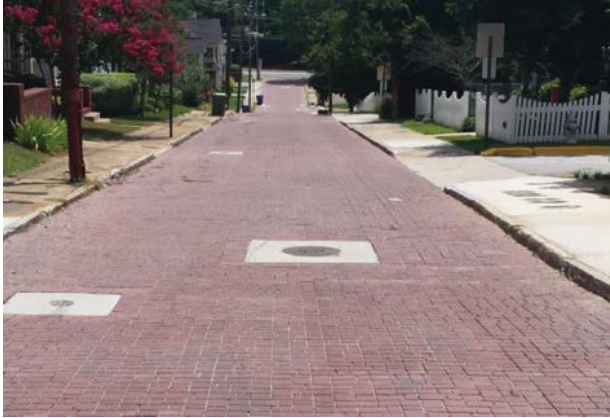
Permeable pavers used for low-speed roadway
