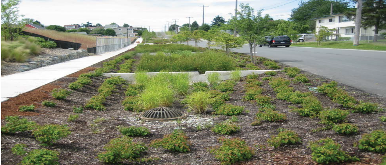
Bioswale (Credit: Kentucky Water Alliance)
