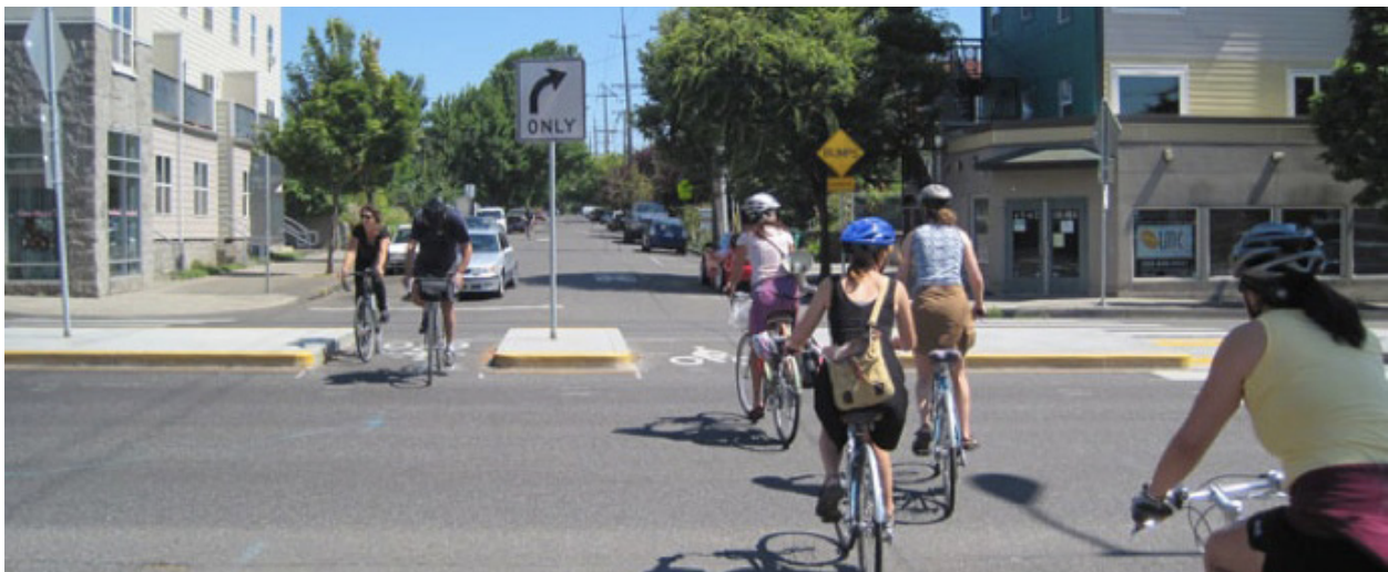
Median refuge island used in the streets of Portland, OR. (Credit: National Association of City Transportation Officials)
