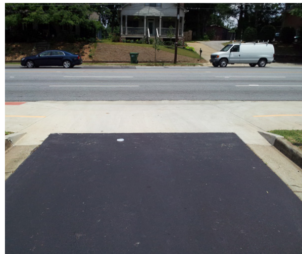
Good integration of driveway apron and sidepath
