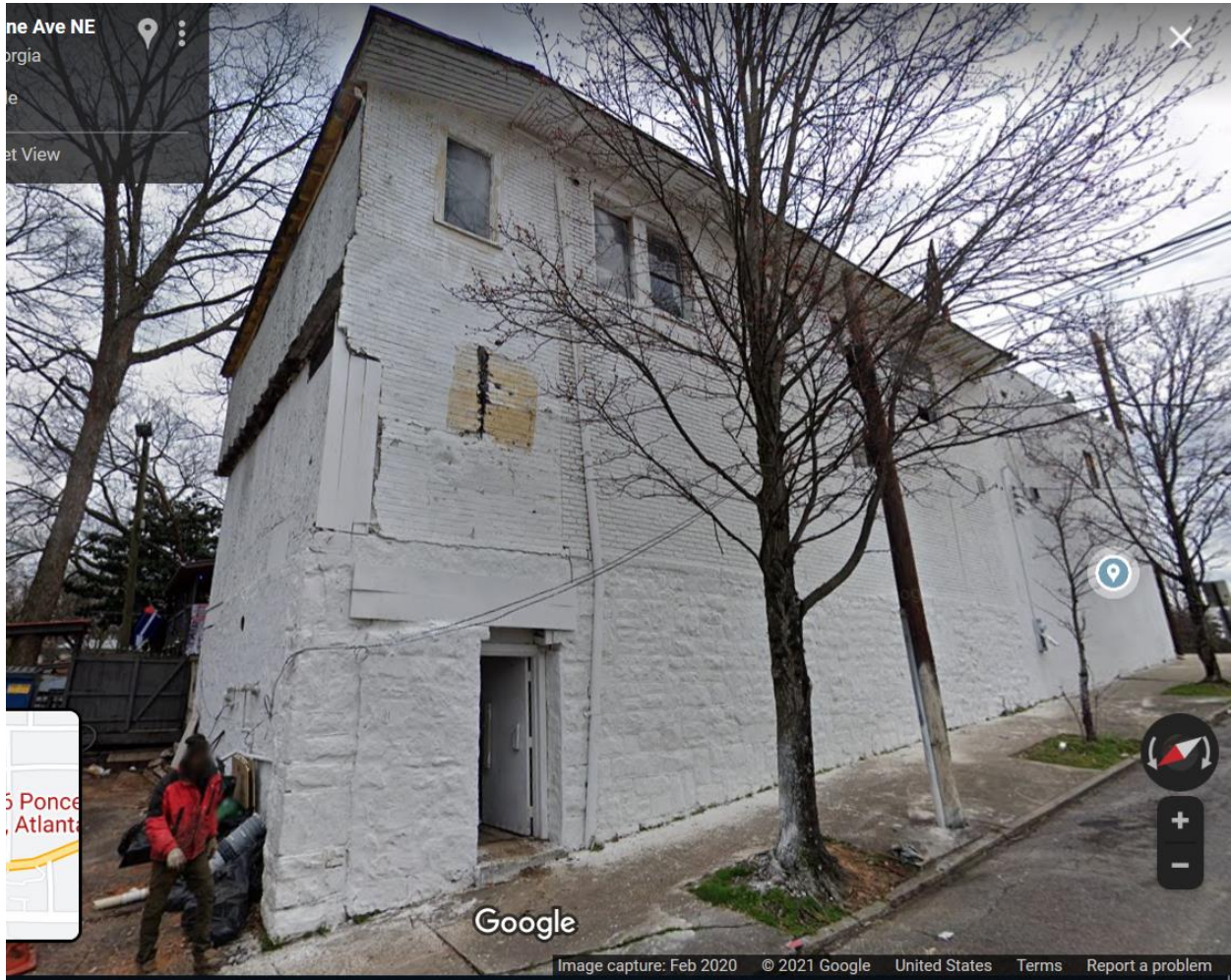
Google Streetview Image – February, 2020 – looking southeast at Argonne Avenue (west) façade
